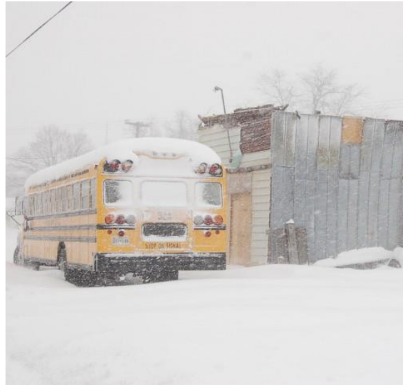
February 10, 2010 - A school bus sits Wednesday on Denton's Gay Street next to a two-story shed, the roof of which collapsed earlier in the day under the weight of fallen snow and ice. Caroline County officials said no was injured when the roof caved in.
