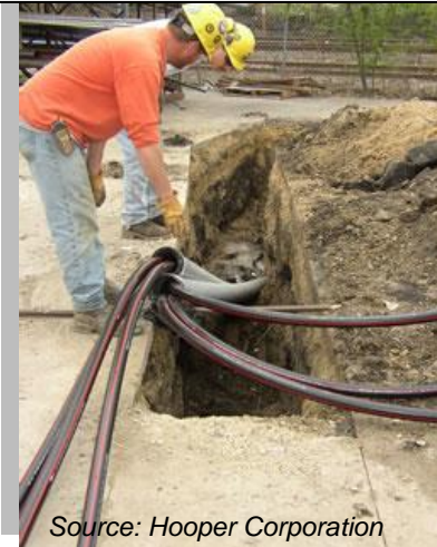
Installation of Underground Power Lines
