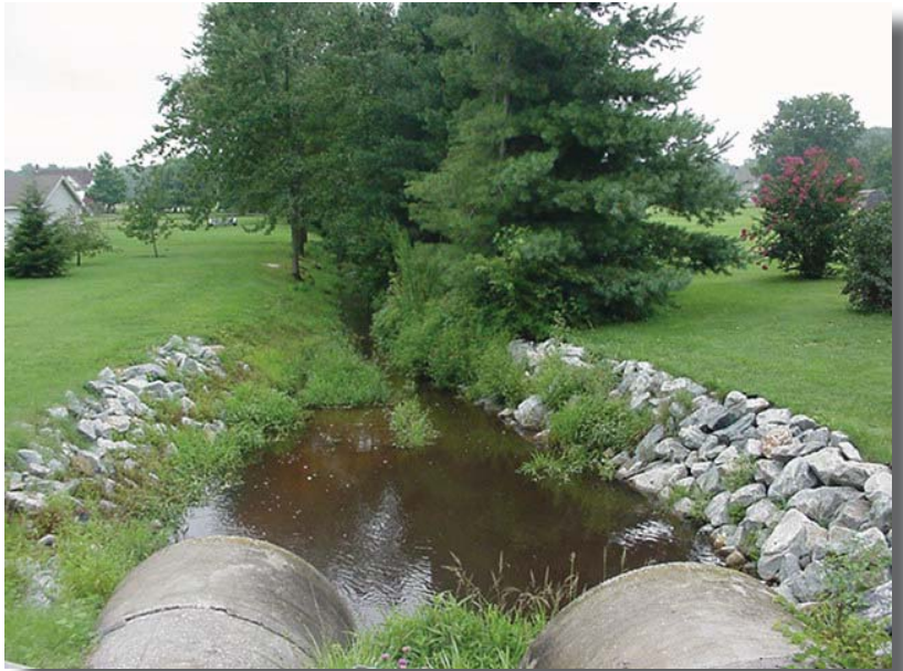
Stone is one of many BMP bank stabilization methods used to prevent blow-outs and channel obstructions for PDAs. Photo courtesy of the Caroline County SCD.
