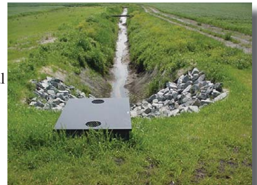
Longmarsh PDA with BMP installed. Water control structures are built across drainage ditches to prevent gully erosion, reduce nutrient loadings, and maintain proper water table levels. Photo courtesy of Caroline County SCD.
